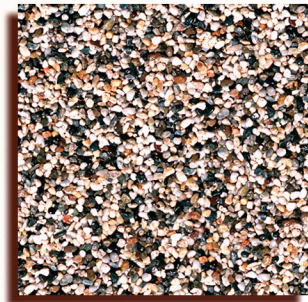
Exposed Agregate Crosswalk Paving
