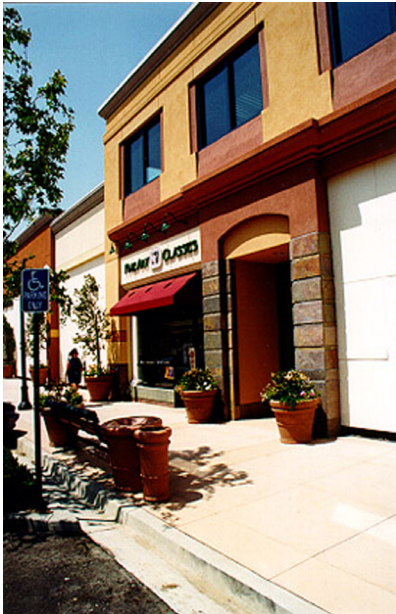
Cornice detail helps to differentiate first and second floors.
