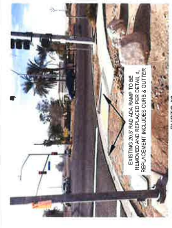
PHOTO #6 NORTH-WEST CORNER - Labrucherie Rd & Aten Blvd Intersection EXISTING 20.9' ADA RAMP TO BE REMOVED AND REPLACED PER DETAIL 4. REPLACEMENT INCLUDES CURB & GUTTER.
