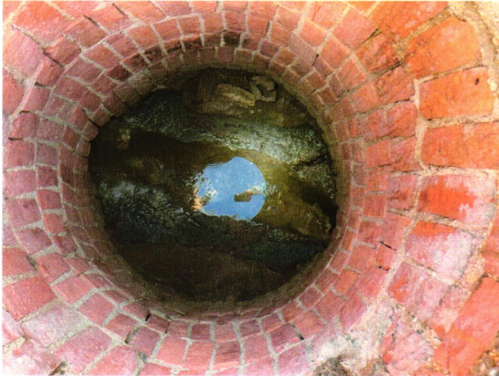
View within MH #42 to be rehabilitated.
