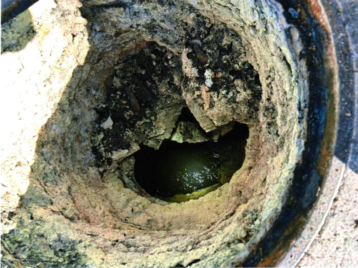
View within MH #348 to be rehabilitated.
