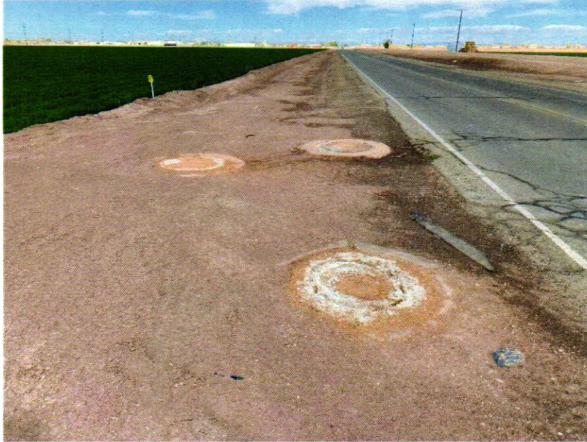
Manhole #359 (located in foreground) and two unnumbered manholes to be removed. View north on the western side of Clark Road.
