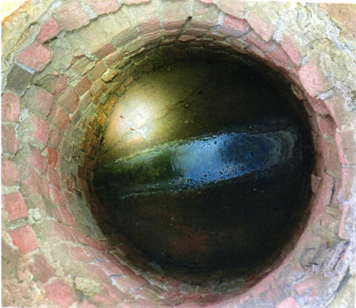
View within MH #55 to be rehabilitated.
