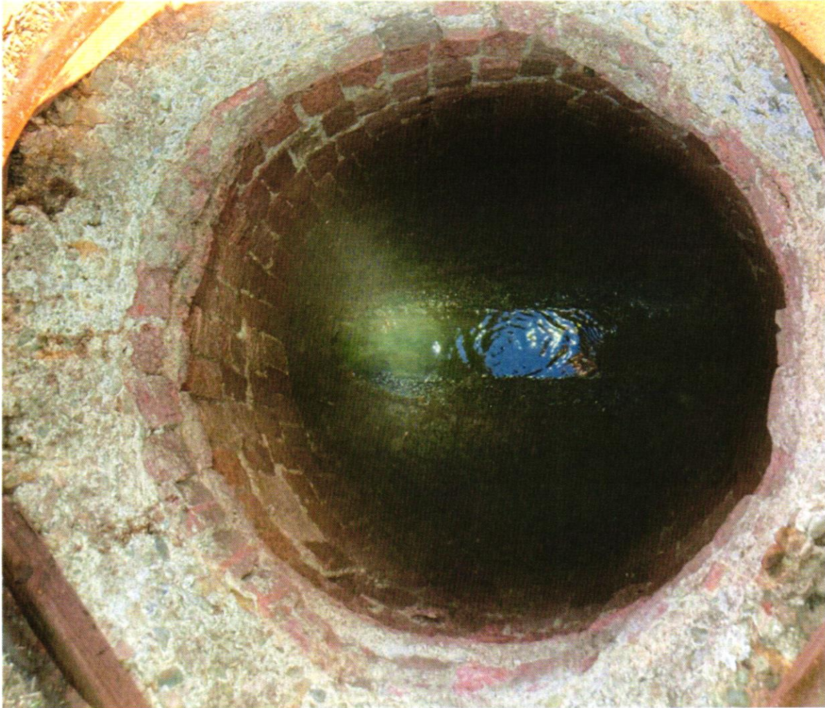
View within MH #59 to be rehabilitated.
