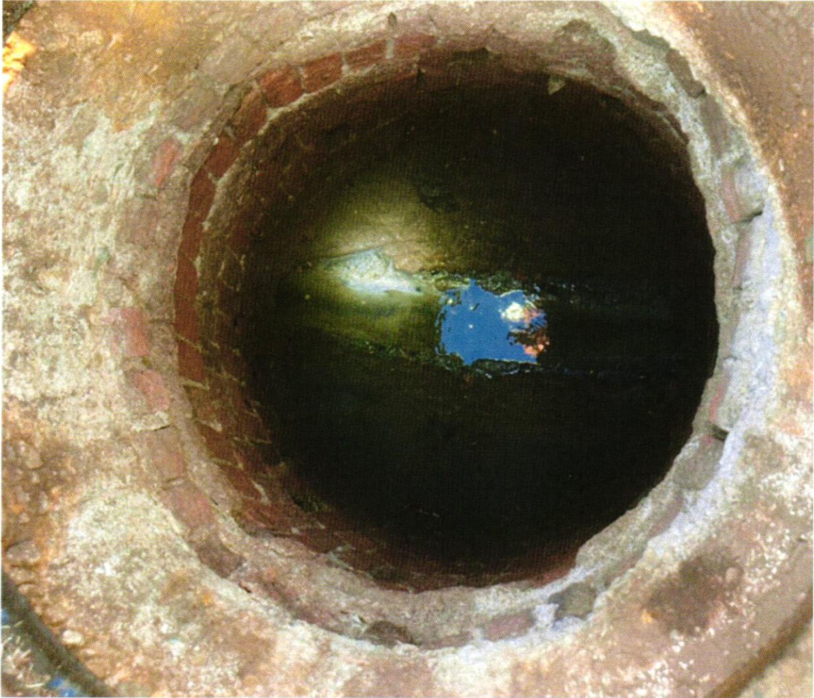
View within MH #58 to be rehabilitated.
