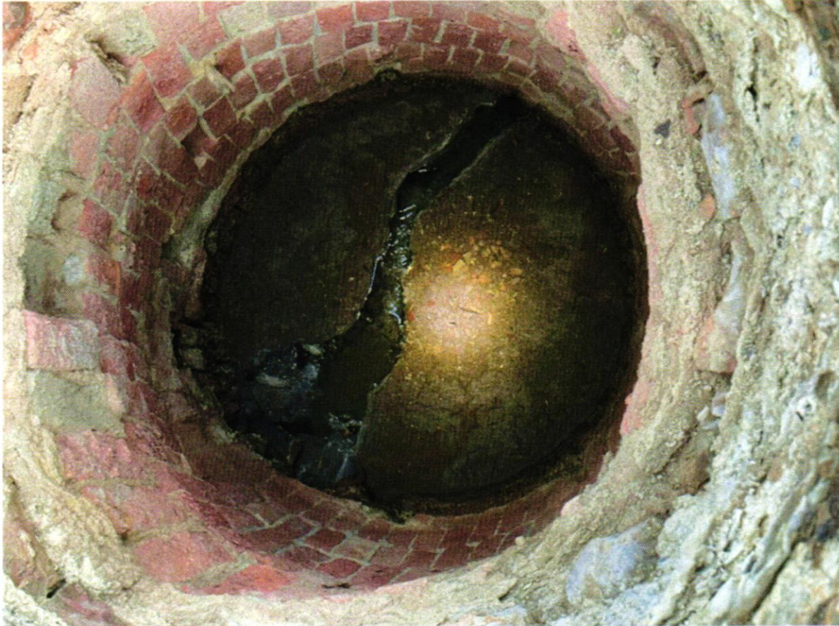
View within MH #51 to be rehabilitated.
