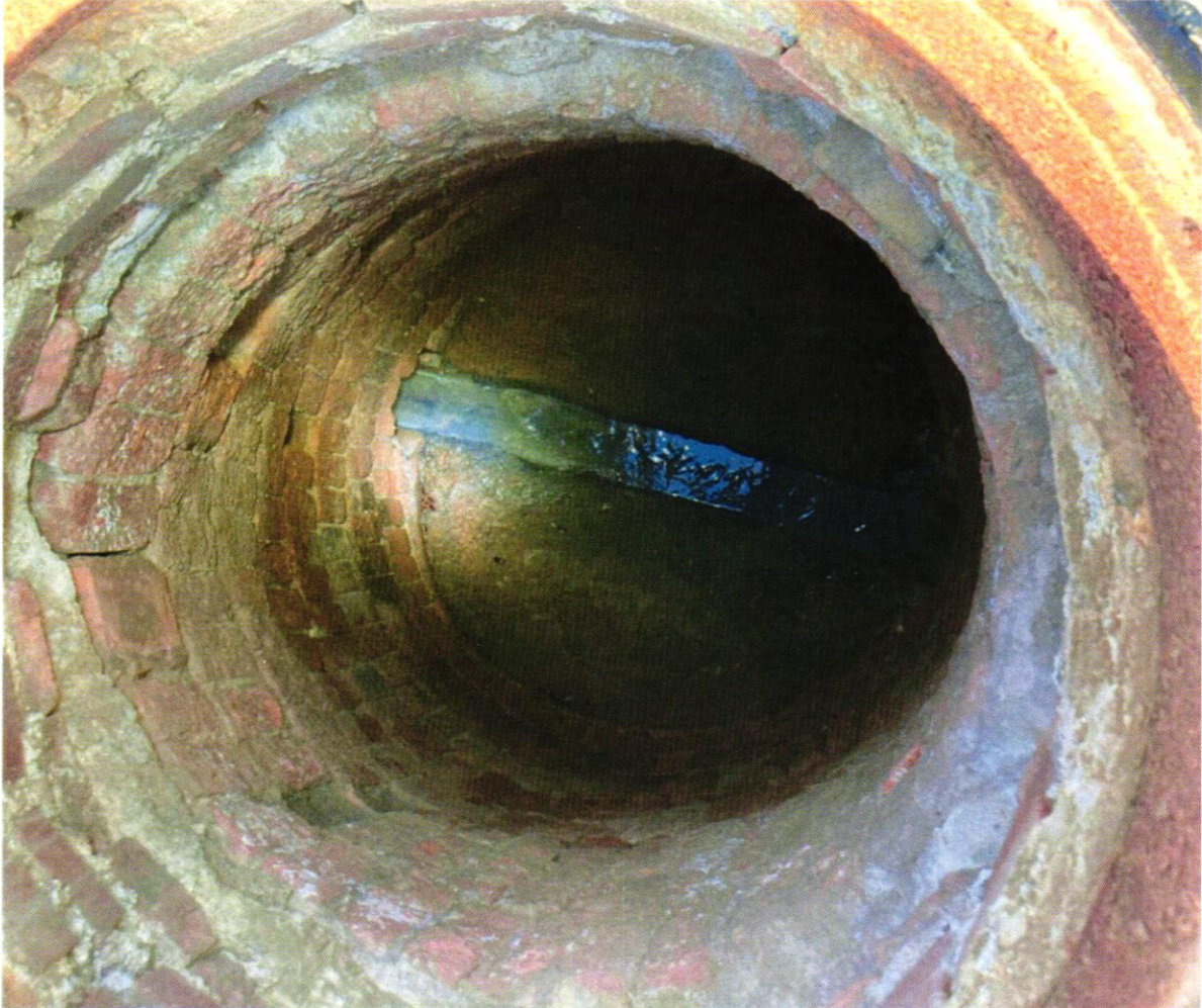
View within MH #60 to be rehabilitated.
