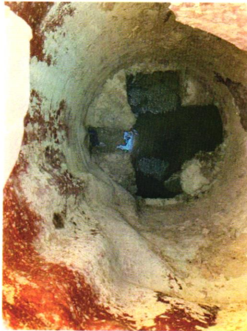
View within MH #1142 to be rehabilitated.
