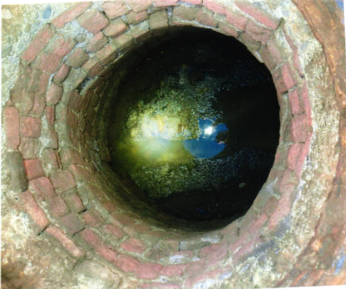
View within MH #56 to be rehabilitated.
