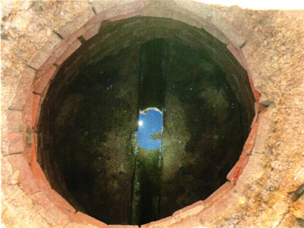
View within MH #28 to be rehabilitated.
