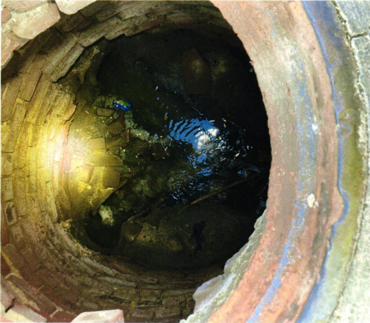
View within MH #54 to be rehabilitated.
