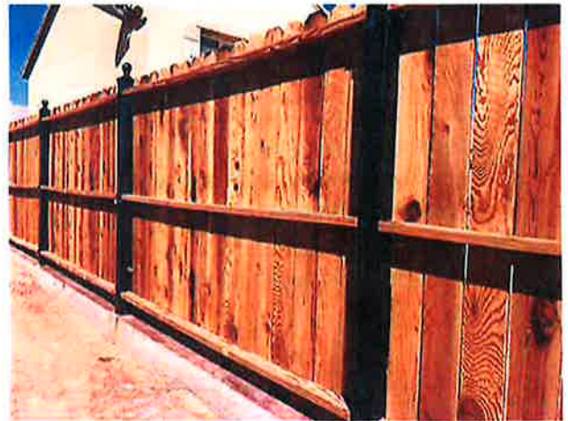
Ornamental Iron and Wood Fence
