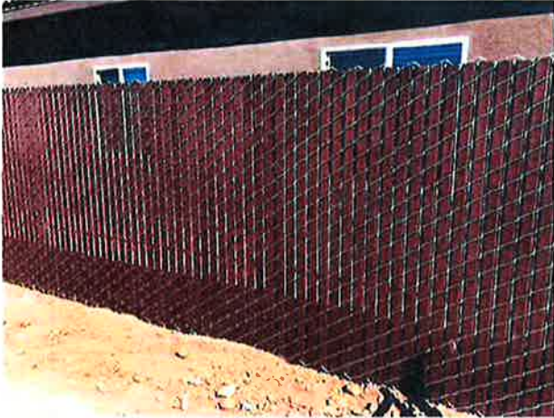
Privacy Chain Link Fence
