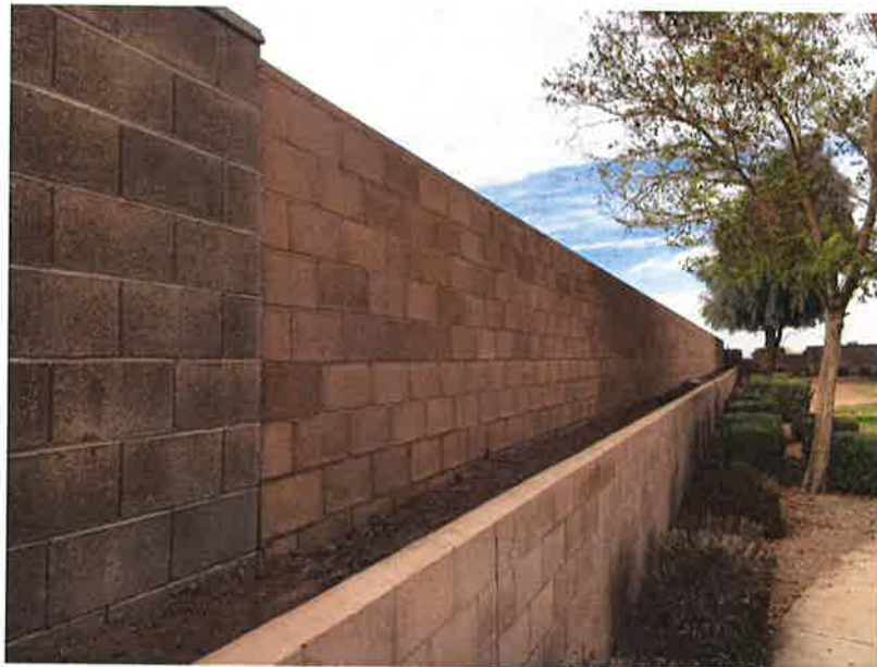
SKY RANCH CONCRETE MASONRY WALL PROJECT COMPLETED FEBRUARY 6, 2019
