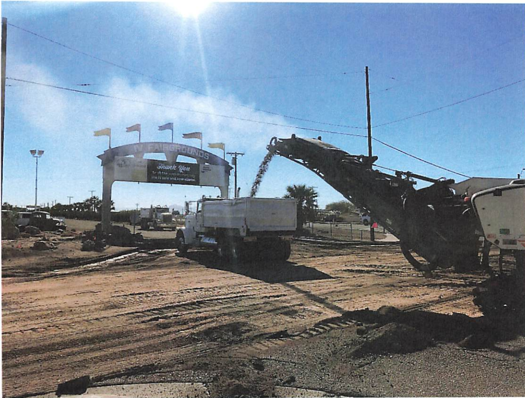
Project Site During Construction Phase.
