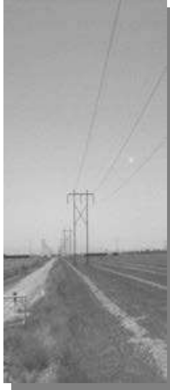
Central Drain running east/west on the southern boundary
