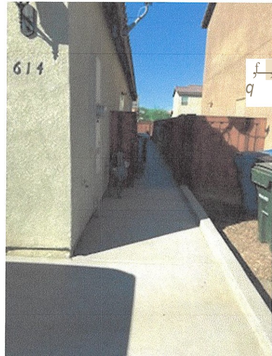
East Side of Preciado Residence
