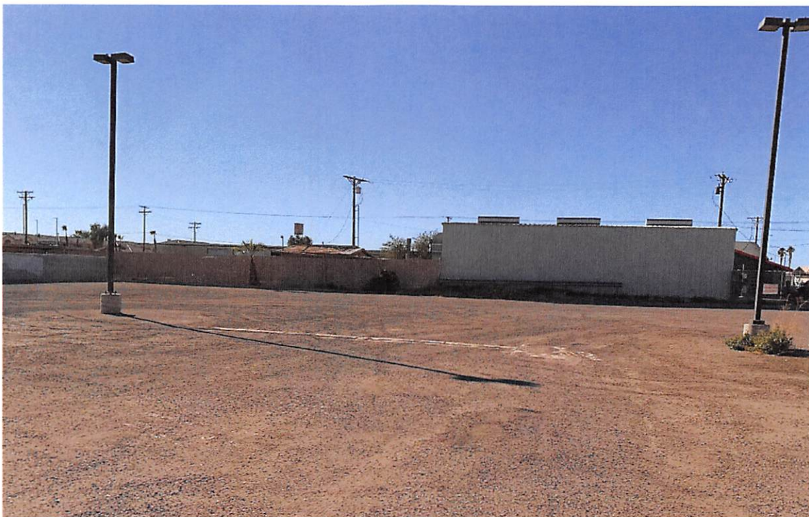
PARKING LOT AND LIGHTING
