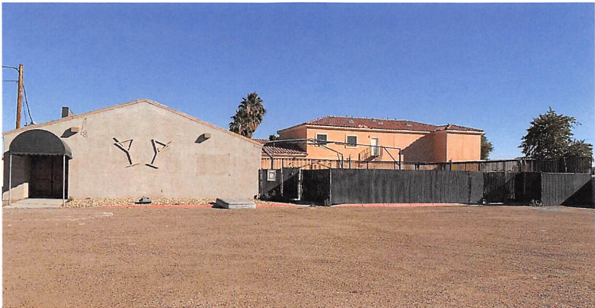
BACK VIEW OF ENTRANCE AND PATIO
