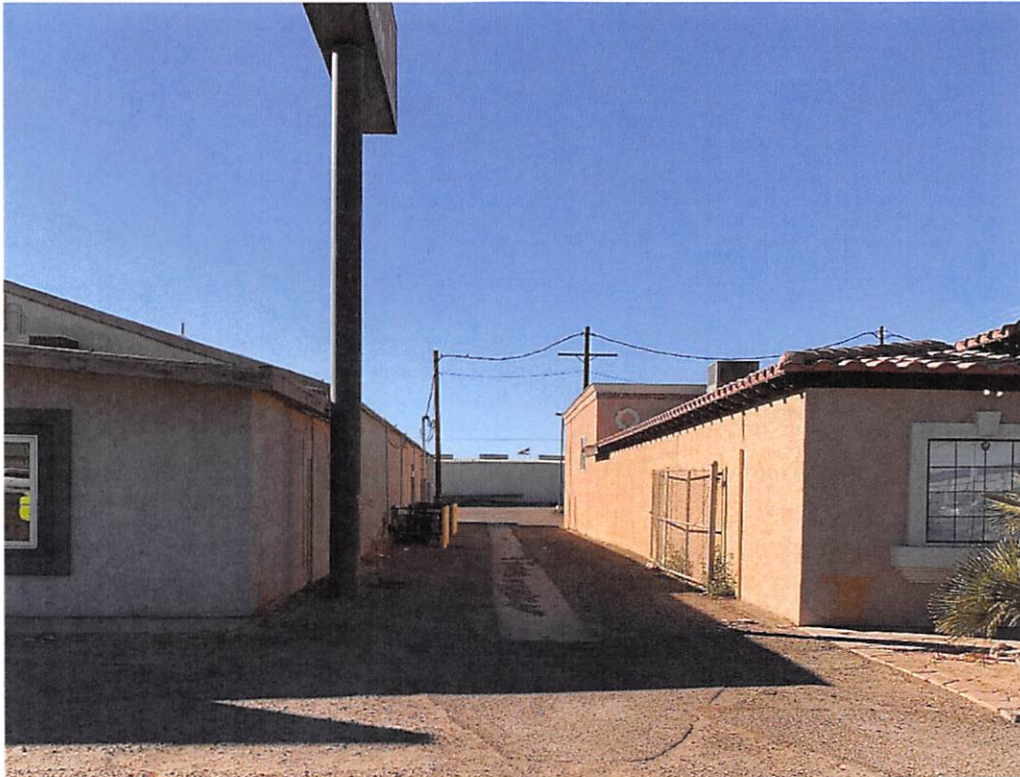
FRONT EAST ENTRANCE
