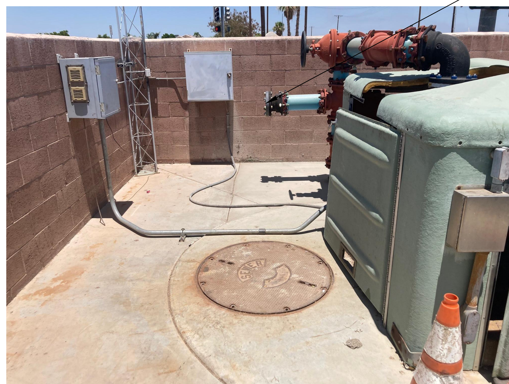
VIEW NORTH WITHIN CROSS STREET LIFT STATION
