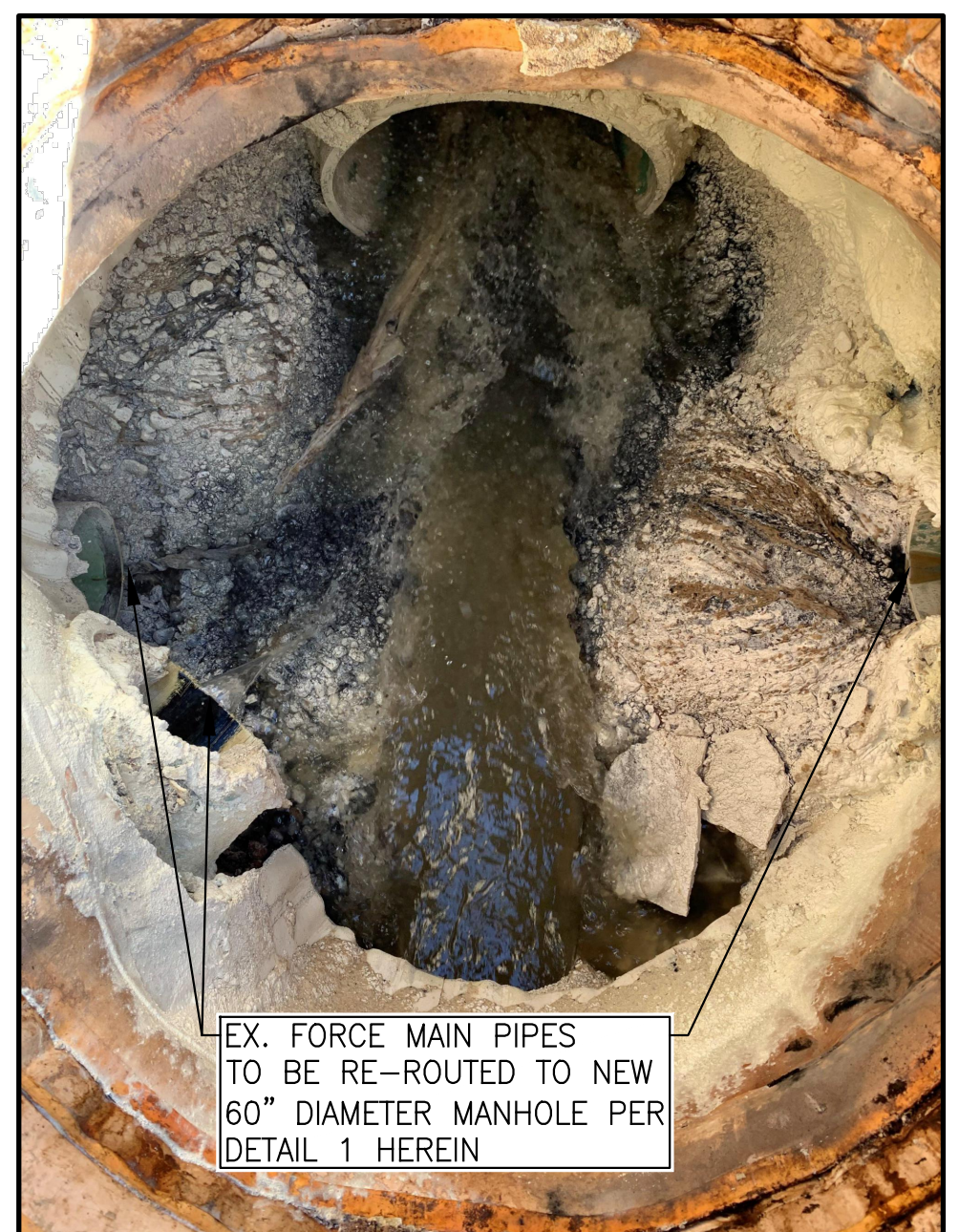
VIEW NORTH WITHIN EXISTING MH #359 TO BE REMOVED
